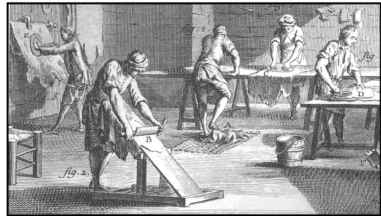
After hides were cured in pools with tannin, the leather had to be curried—impregnated with oil or grease—and readied for the use of the bootmaker or harnessmaker or other craftsman. The figures in this drawing show various stages of oiling and scraping the leather with a variety of knives, combs, and buffers.
