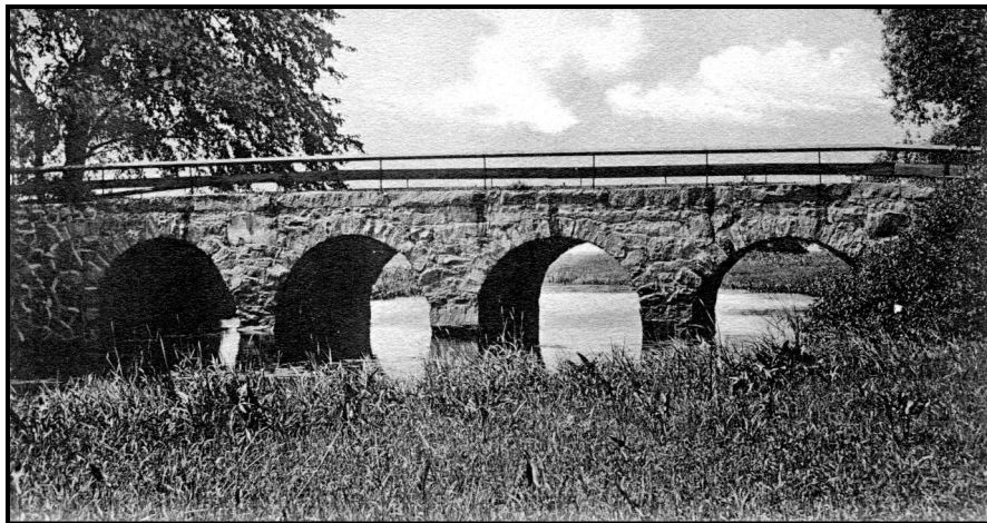
The first cart bridge in Sudbury over the river was built at this site about 1642—reportedly the first frame bridge in Middlesex County. This four-arch stone bridge replaced a wood bridge in 1848.
